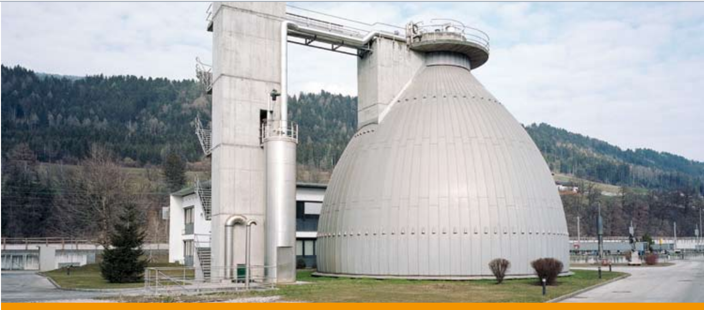
Solids separated from the used cooking oil are fermented with other waste to produce methane for two 300 kW gas engines
