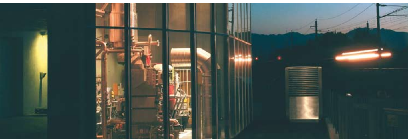
The attractive Fritzens power house resembles a boat
