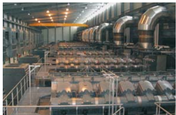
18V48/60B supplying 18 900 kW each
