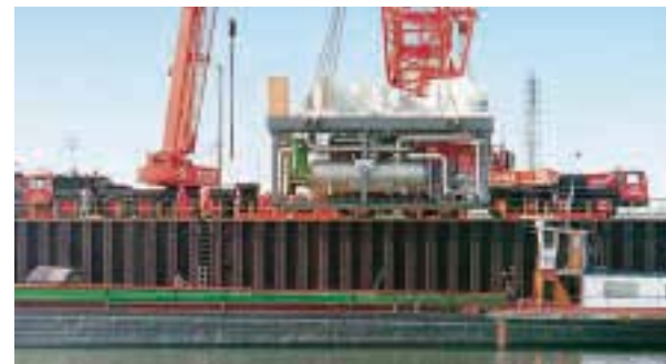
Transport of the compressor package to the site
