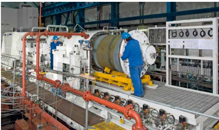
MAN Diesel & Turbo compressor type RB on testbed
