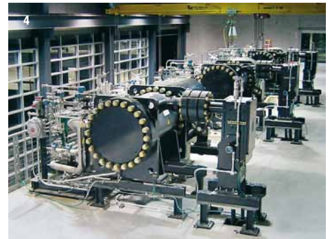
4 The first three HOFIM™ Sealed units operating in a gas storage facility in the USA. The plant layout allows the three units to operate in parallel, but also two units in parallel, feeding the third unit in series for high-pressure ratio requirements. Each motor is rated at approximately 7 MW. Gas can be compressed from 55 up to maximum 220 bar.
